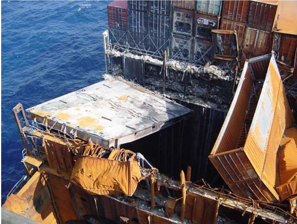
Photo 10. The aftermath of the Nov 15 th explosion above hold six. Note the deck hatch (weight approximately 30 tons) that is normally held in place by a series of heavy pins.
