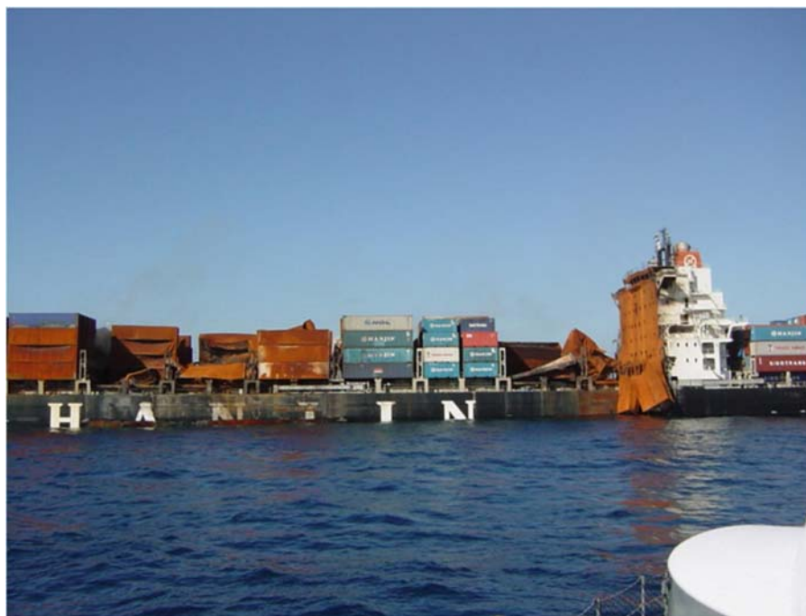
Photo 7. The M/V HANJIN PENNSYLVANIA (port) riding very low in the water as a result of fire fighting efforts. Note the burned containers above hold three and the missing and burned containers above hold four. Also note the raised and twisted deck hatch, the missing containers and heavy damage to the containers above hold six forward of the accommodation. Damaged containers above hold six are hanging over the port side
